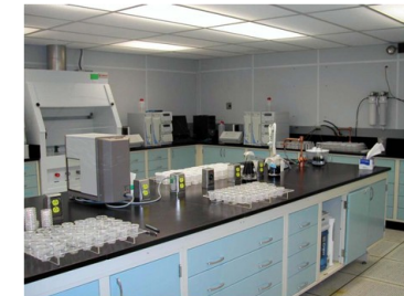
Class 100 Clean Room facility
